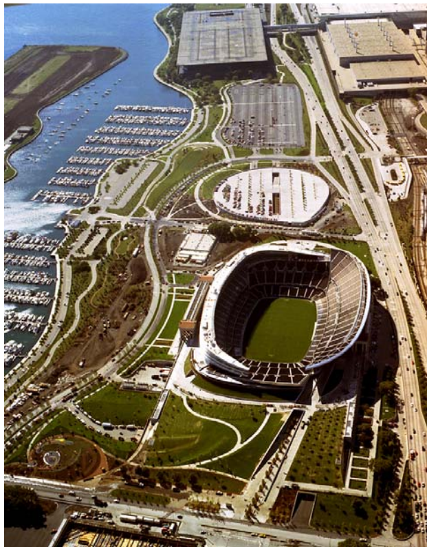
Soldier Field Renovation at North Burnham Park, Chicago, Illinois JBC Soil & Irrigation Consultants
