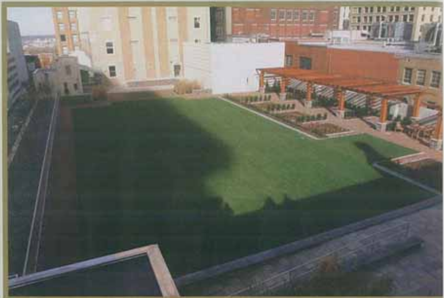
Sustainable design elements at 915 Walnut in Kansas City, Mo., include a roof garden supported by an engineered additional pre-cast double-T support and regionally harvested IPC pre-cast materials.
