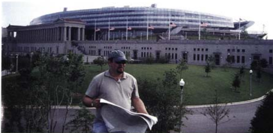
The landscaped rise behind Bruce serves as the roof to a 2,500 vehicle underground parking garage.
